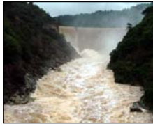
Slab Creek Dam at flood stage, South Fork American River.
